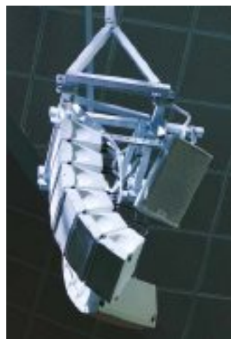
The church's left Nexo Geo M6 cluster with arrays for the house and side-fill, and a rear-mounted PS10 for stage monitoring
