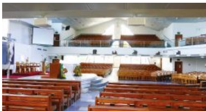
Nexo ID24i loudspeakers serve as fills beneath the gallery
